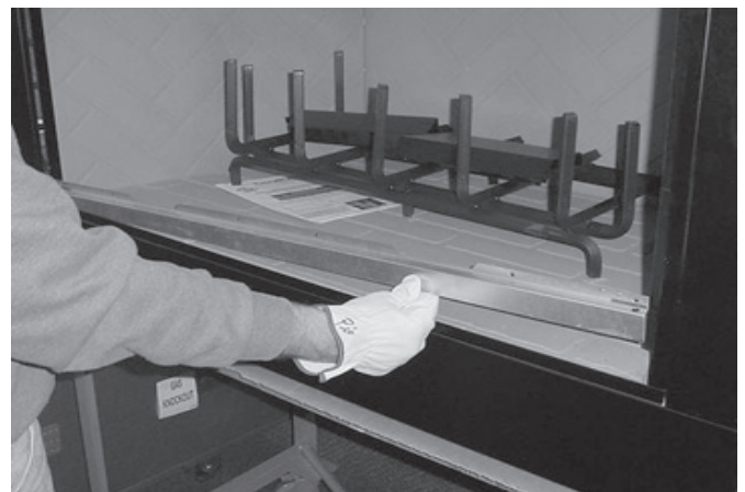
Figure 1 - Install the Door Track
