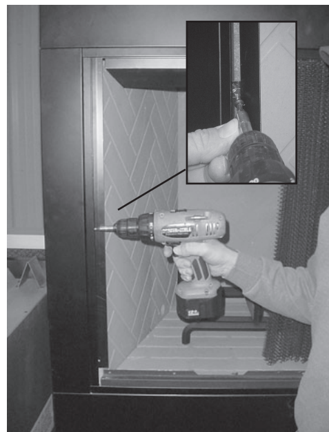
Figure 5 - Fastening the Side Filler
